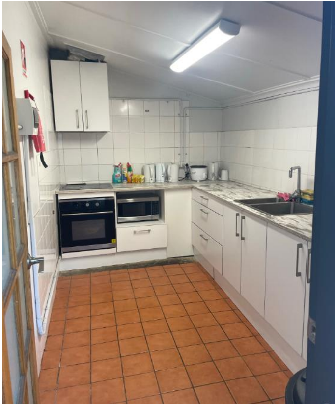
Figure 6: Existing skillion addition comprising communal kitchen which is proposed for demolition
