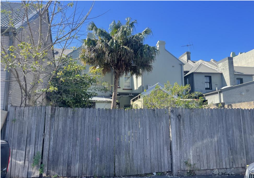
Figure 9: View of the rear of the site from Little Mount Street, subject site is the green terrace on the right-hand side
