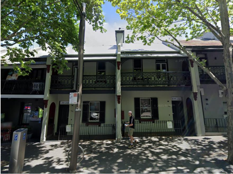
Figure 2: View of terrace from Harris Street, the subject site is the green terrace located on the left-hand side
